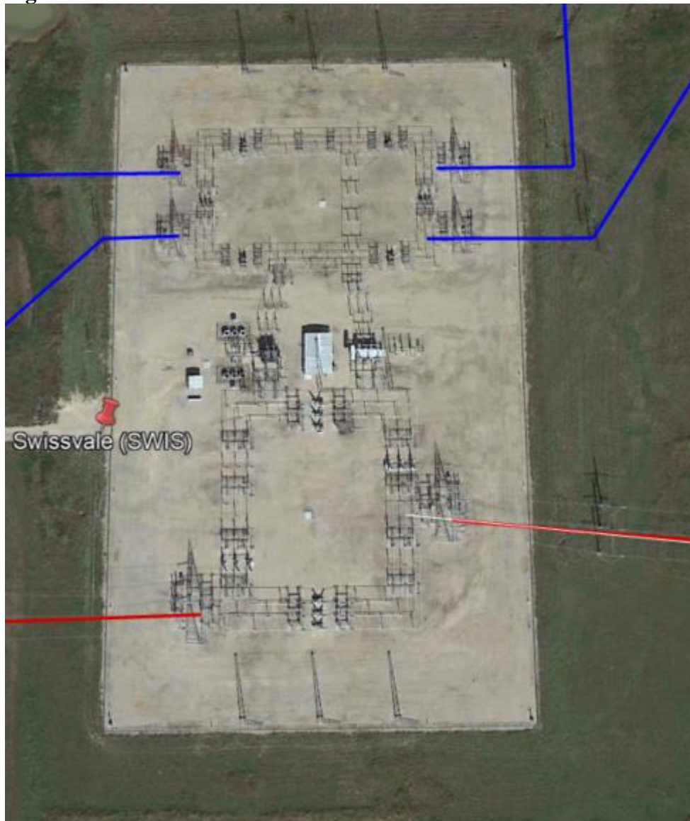
Figure 25 – Swissvale 345kV Substation
